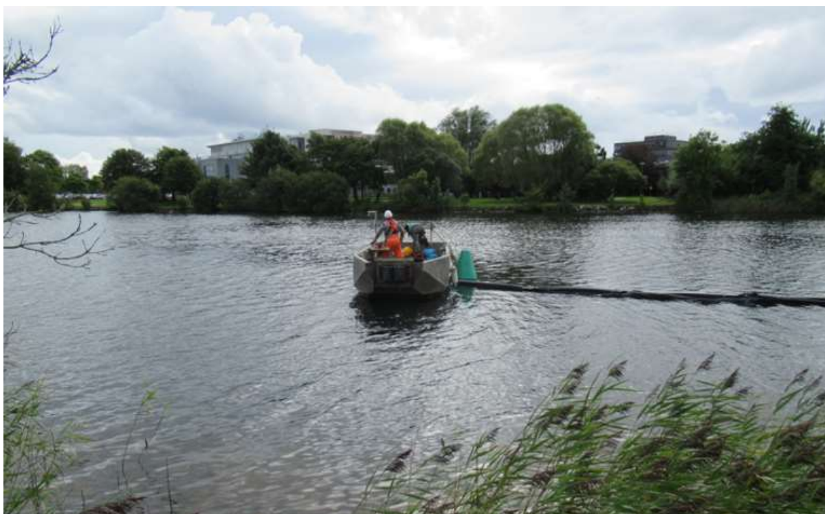
Figure 3-85: Installation of a silt curtain in the River Corrib, Co. Galway
