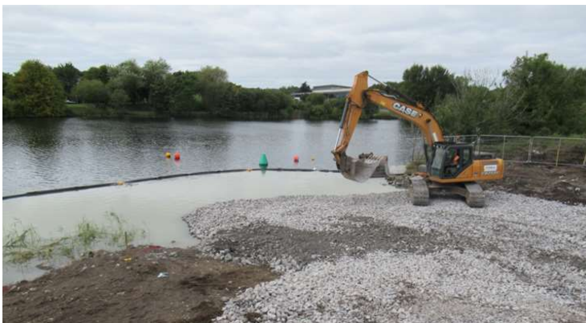
Figure 3-86: Silt curtain retaining contaminated water during advanced works for sheet piling
